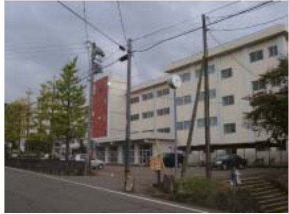
Photo 3. General view (T-1 building of T-High school)
